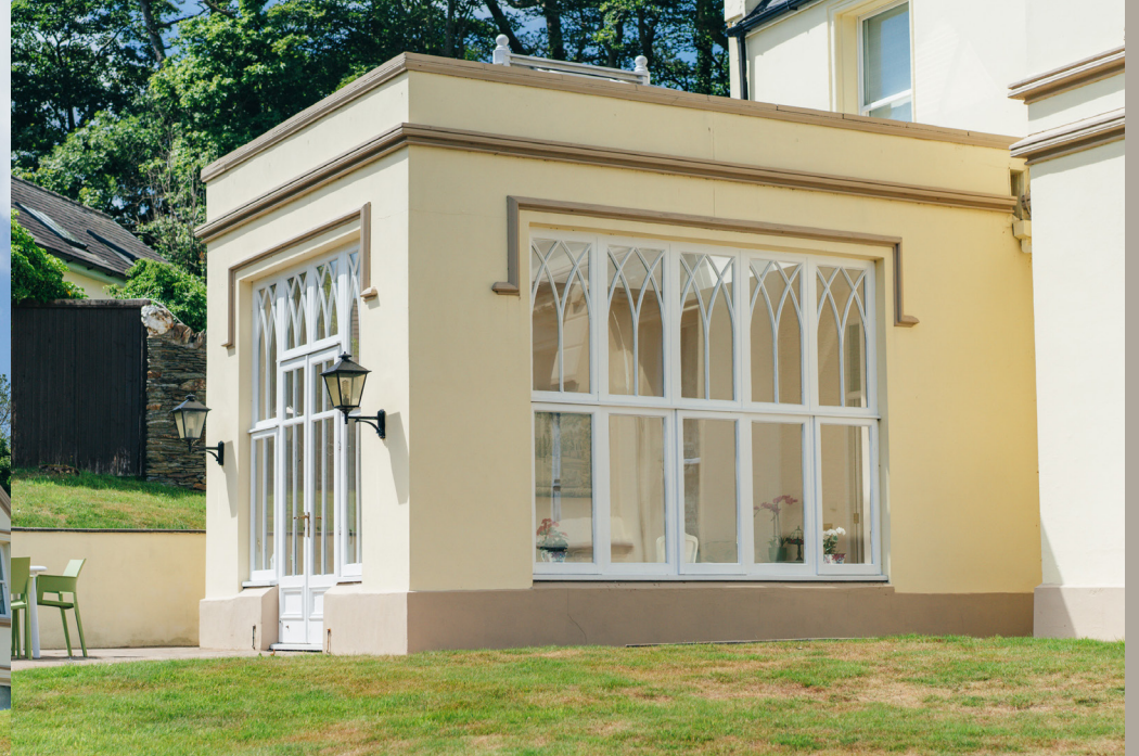
SUN ROOM EXTERIOR
